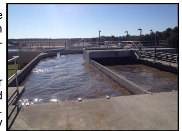
Waste taking a 4 million gallon microorganism bath.
